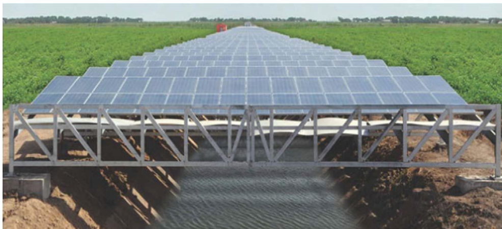
Fig. 4. Canal top solar systems.
